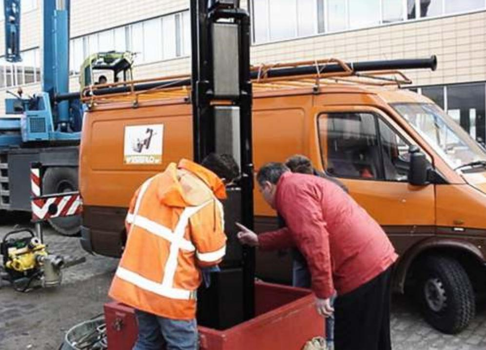
Inspection of a GeoThermic system by Westerlo, in the Netherlands. SWEP B45 BPHEs being lowered into the drilled well.
