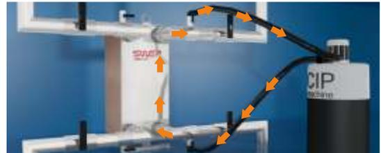
Connect the CIP machine via inlet/outlets on front or back. Pump the solution into the BPHE using the lower connection to expel air. Reverse the flow direction every 30 minutes.
